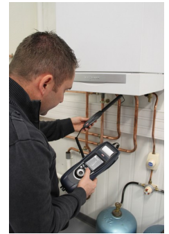
Ambient CO checking
